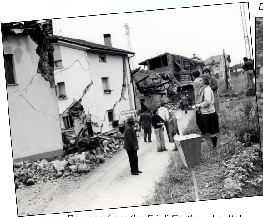
Damage from the Friuli Earthquake, Italy
